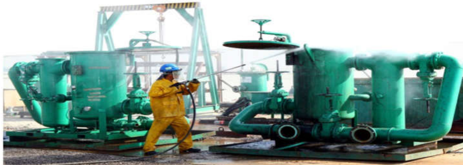
Boiler and Heat-Exchanger tube cleaning using environmental friendly methods.
