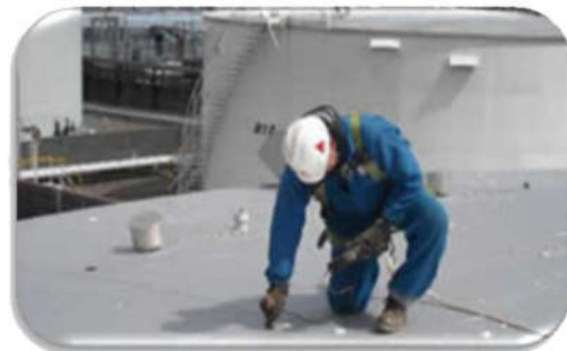
Manual UT inspection on tank top
