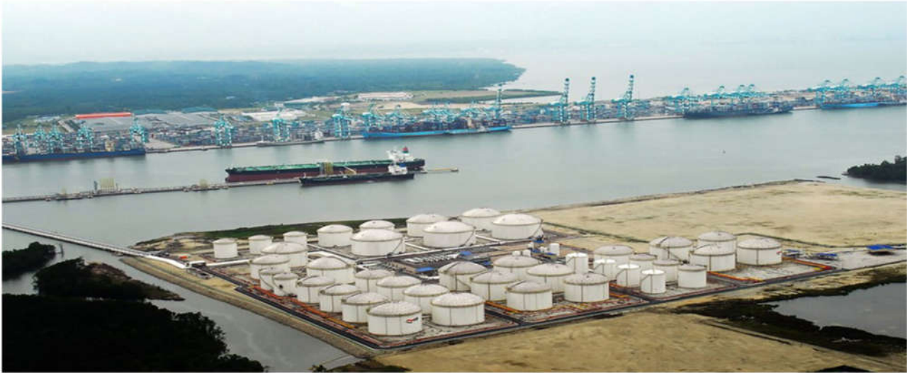
Tank Fabrication and Erection.
